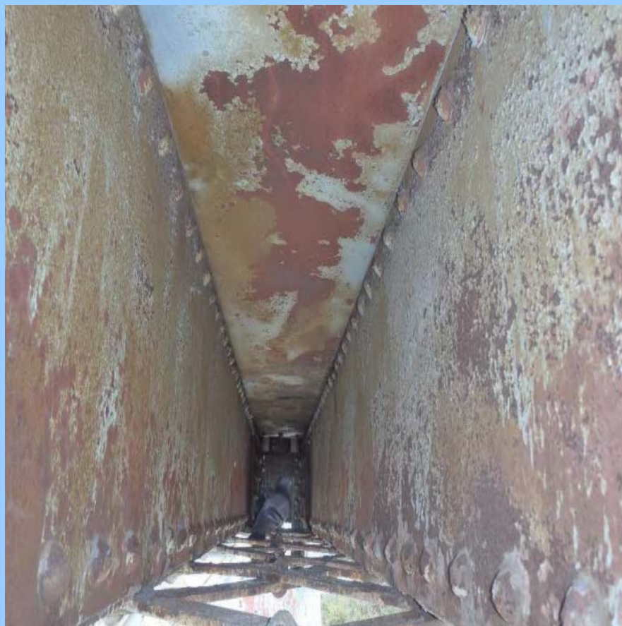
Typical localized material loss and heavy pitting in north truss members
