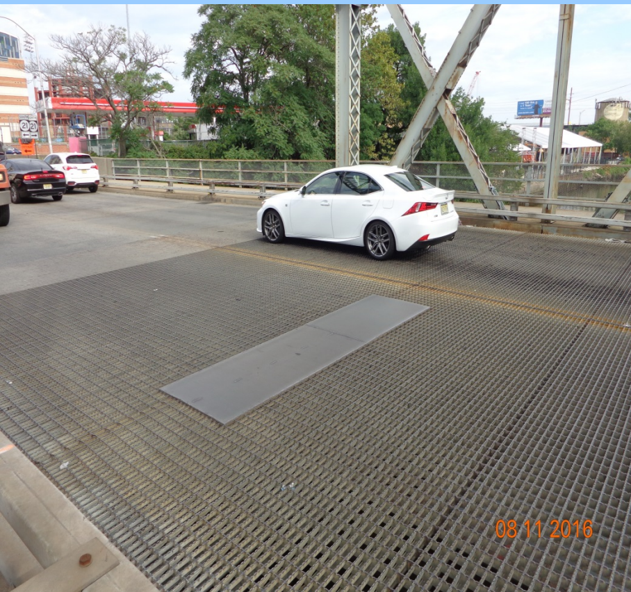
Steel deck grating in swing span
