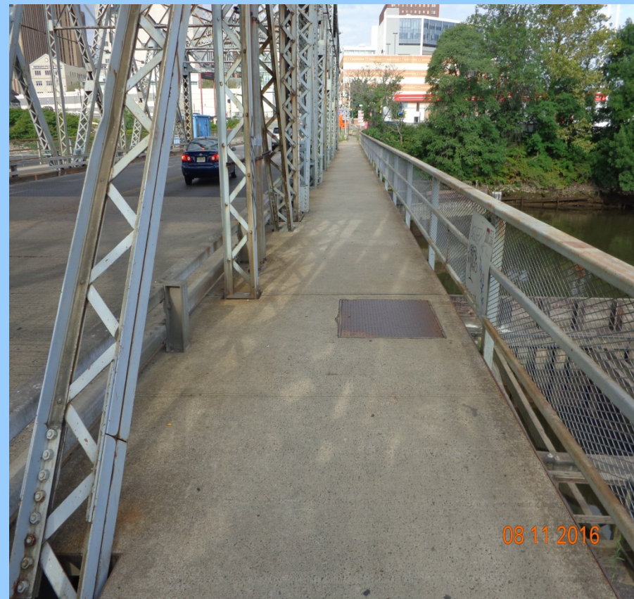
Substandard bridge railing (typical)
