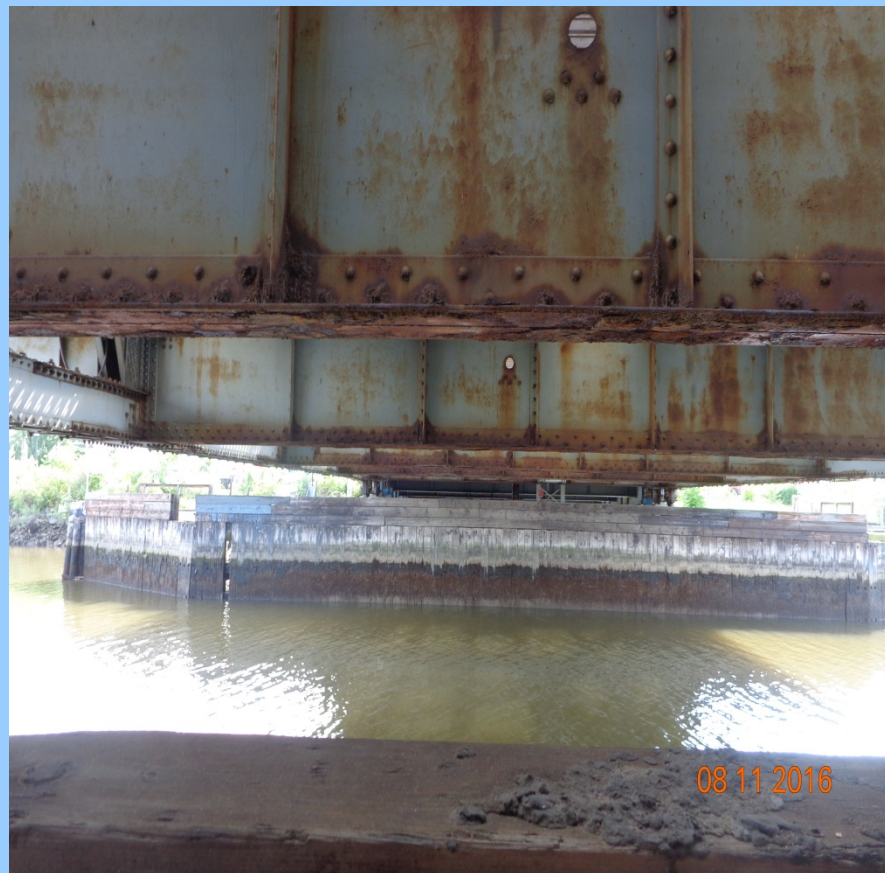
Section loss and heavily corroded floor beams in swing span
