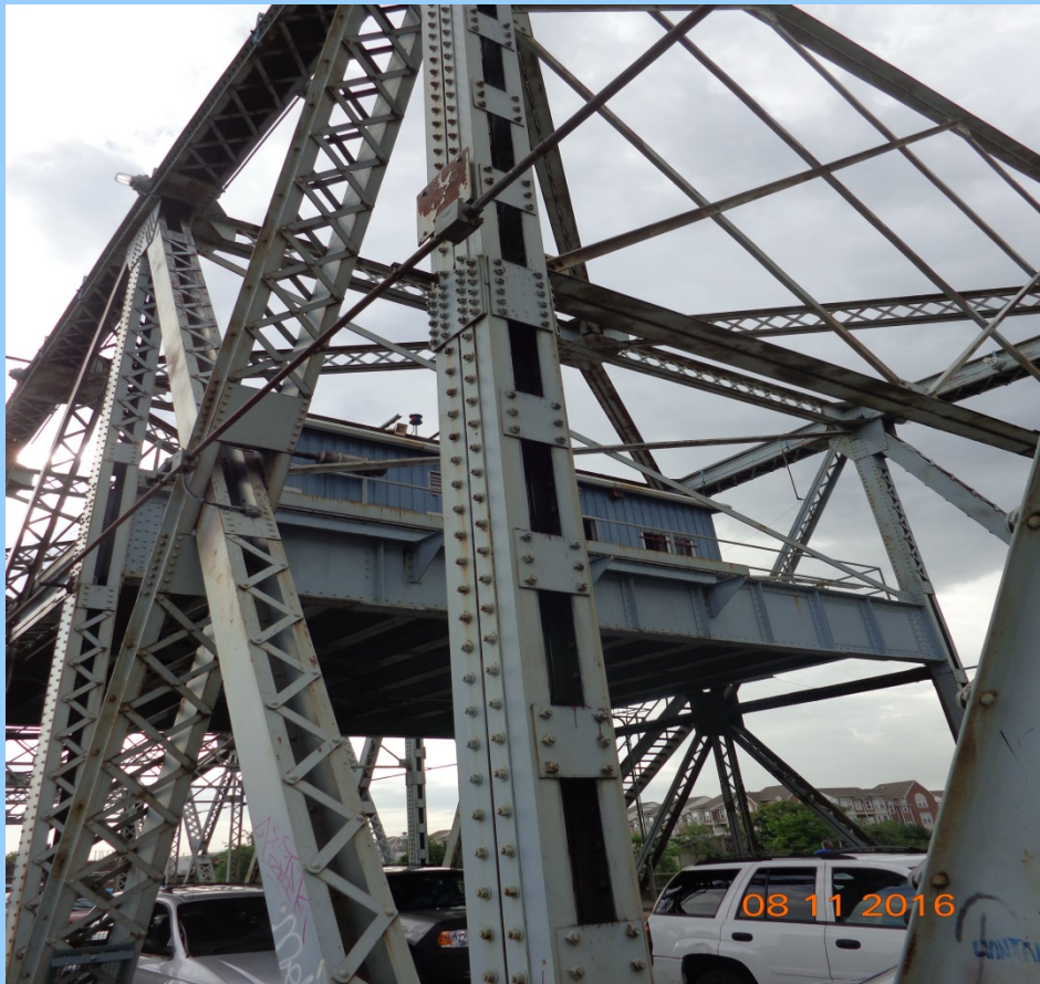
Rusting of gusset plate in truss leg
