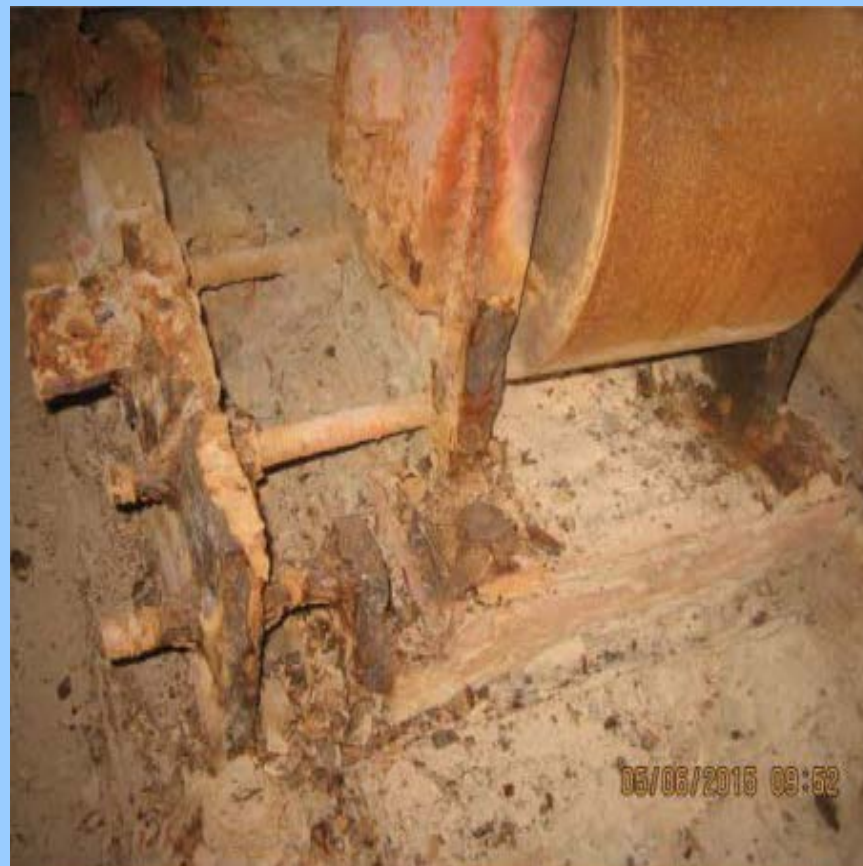
Heavy corrosion and section loss of tapered roller support
