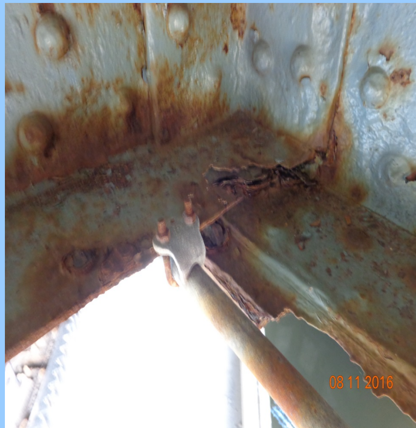
Localized section loss of floor beams and stringers in swing span
