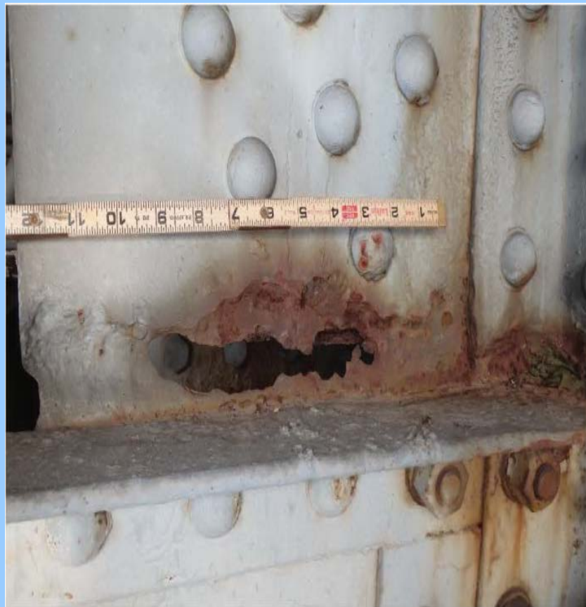
Section loss of gusset plate in south truss at east swing
