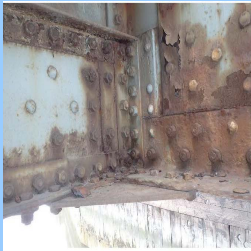
Severely corroded and deteriorated floor beam web and bottom flange in the south truss west swing span
