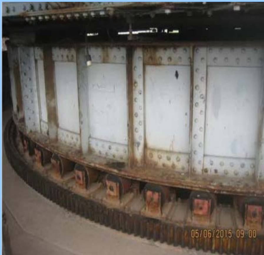
Drum girder and tapered rollers
