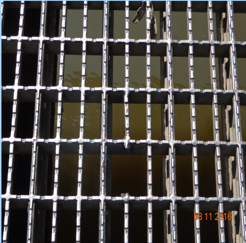
Steel deck grating in swing span
