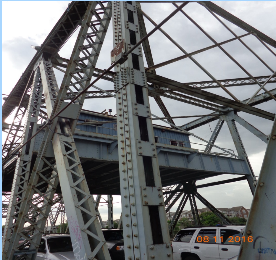
Rusting of gusset plate in truss leg
