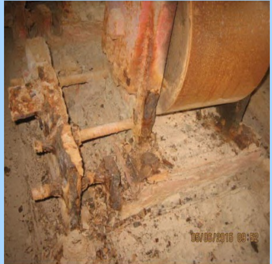
Heavy corrosion and section loss of tapered roller support
