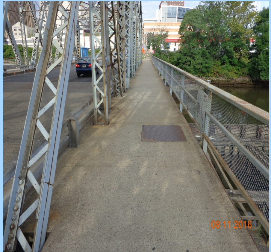
Substandard bridge railing (typical)
