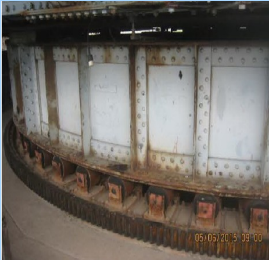
Drum girder and tapered rollers
