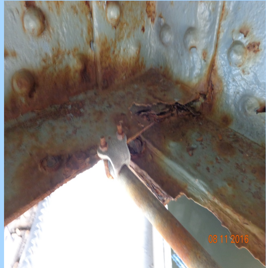
Localized section loss of floor beams and stringers in swing span
