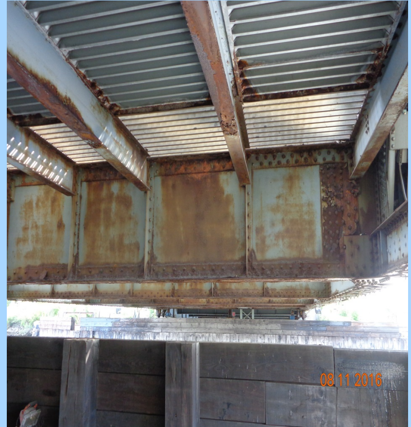
Localized section loss and heavy pitting of floor beams and stringers in swing span
